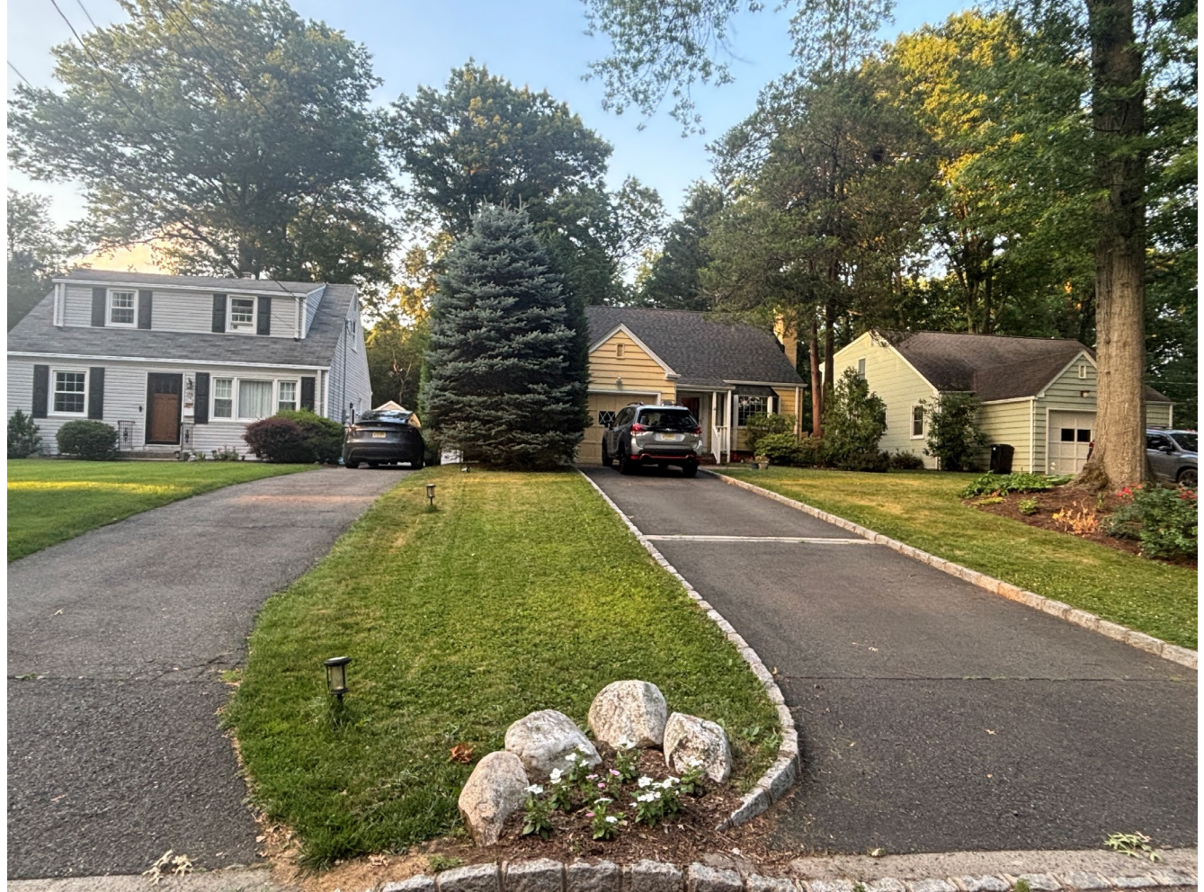
Front view of 174, 170 and 164 Russell Road
