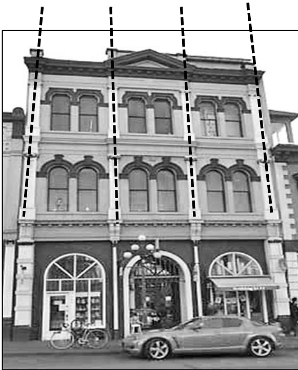
Vertical articulation using column piers and windows at equally spaced intervals.
