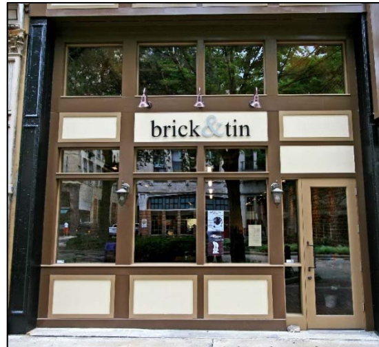
Façade sign with external lighting located above display windows and below transom
