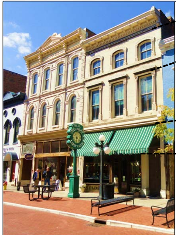
Horizontal alignment of features with adjacent buildings (window sills, cornice lines and trim, awning and transom)
